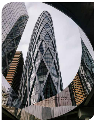
THE TOUR D2 BUILDING IN LA DÉFENSE DISTRICT
